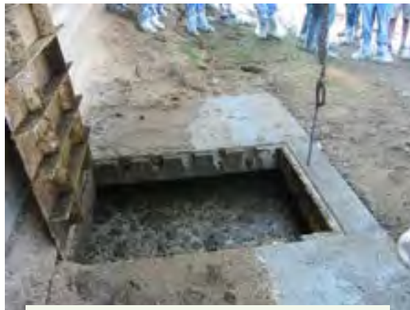
Figure 3.11.a. Manure storage pits are often found below ground level. They are covered until it's time to pump them out. Agitation and pumping release toxic gases. Credit: Penn State Extension Ag Safety Team
