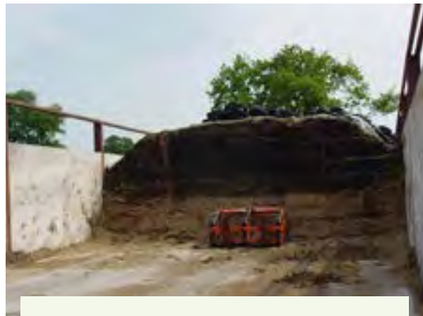
Figure 3.9.1.c. Sight rails offer a visual clue as to how close to the edge of the bunker you are operating the dump truck or packing tractor. These should be kept in good repair. Credit: Penn State Extension Ag Safety Team
