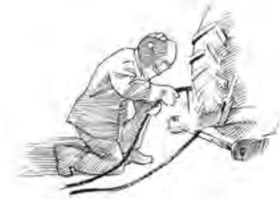
Figure 3.3.a. Welding produces fumes. Illustration by Jeff Mathison.
