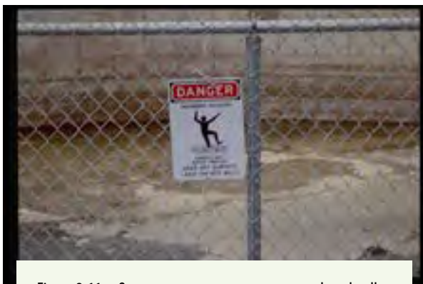
Figure 3.11.c. Open manure storage areas pose a less deadly gas hazard than belowground pits. The major hazard of the open manure storage becomes drowning. Fencing and warning signs alert people of the liquid manure hazard.
