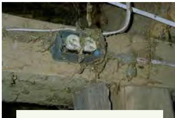
Figure 3.7.c. Dusty, dirty conditions in agriculture contribute to increased fire hazards. What materials in this picture are considered Class A fuel sources? Credit: Penn State Extension Ag Safety Team
