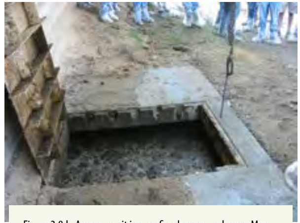
Figure 3.8.b. A manure pit is a confined space work area. Many lives have been lost in manure pits due to toxic gases and lack of oxygen. Credit: Penn State Extension Ag Safety Team
