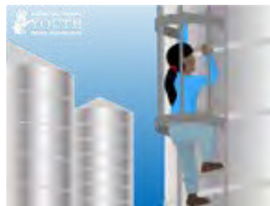
Figure 3.9.c. When climbing silos, use the ladder, stay inside the enclosed protective cage, and maintain a three-point contact with the ladder. Credit: Ag Youth Work Guidelines
